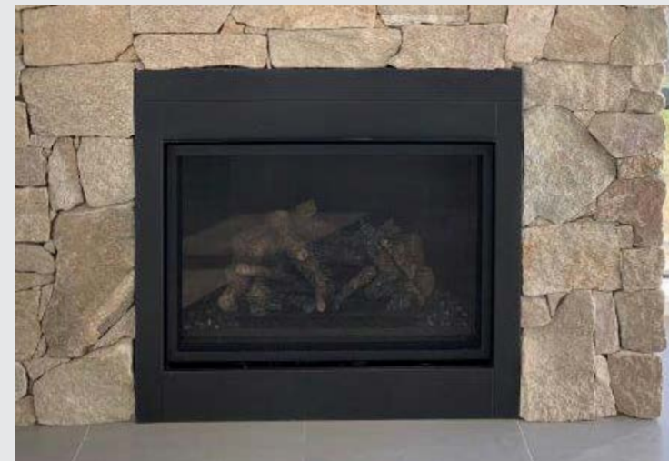
Example of exposed firebox surround (no trim) with stone
